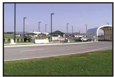
Force protection became top priority after the attacks of September 11, 2001. This leads to construction of new security buildings at depot entrances
